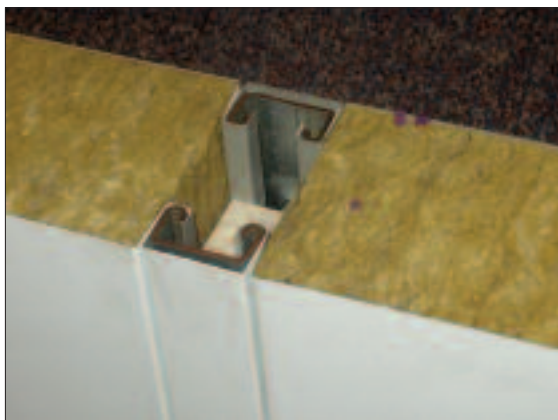
Figure 17: Insulated core panels – internal panel
